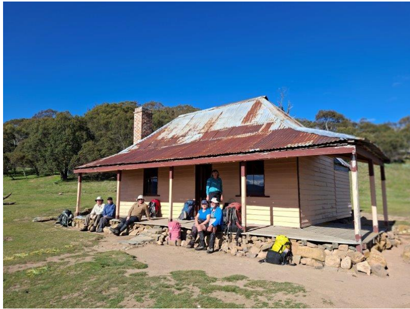
Old Currango Homestead is located just below the tree line at the north west end of Currangorambla Plain, with fantastic views across the plains to the Brindabella Ranges in the east. The primary building was built in 1873 by Tom O'Rourke, who had been grazing on the plain since 1834. It is the oldest remaining building in the Kosciuszko National Park.
